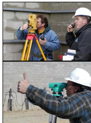
Fig. 13 Monitoring Wall Movement During Lifting Phase
