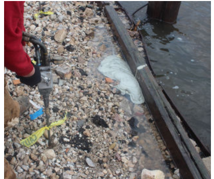
Foam setting up in water. No Chemicals leaching into the water.
