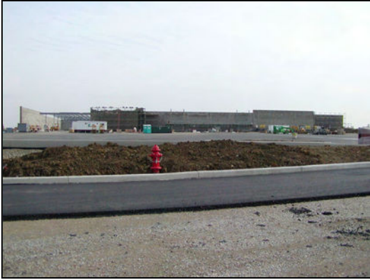
Fig. 6 Distant View of Target Store Site
