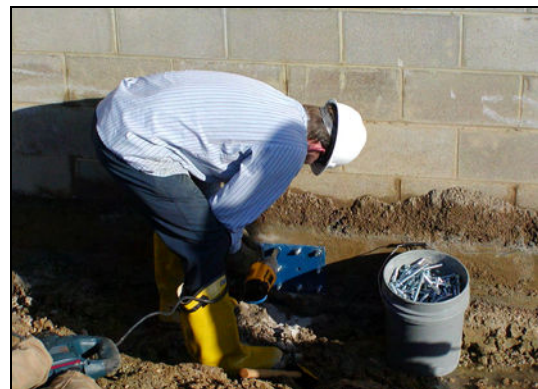
Fig. 10 Bracket Installation
