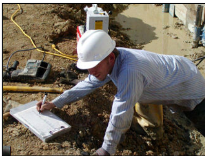
Fig. 12 Logging Pier Depth and Hydraulic Pressure
