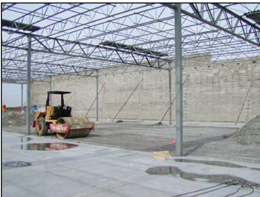
Fig. 7 View from Inside Target Store
