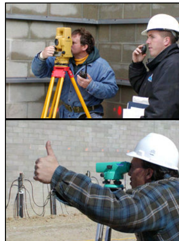
Fig. 13 Monitoring Wall Movement During Lifting Phase
