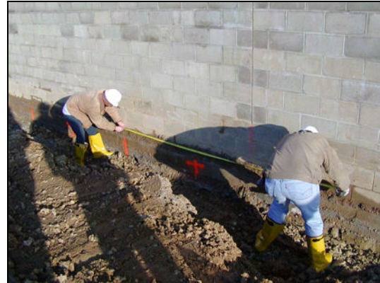
Fig. 9 Marking Bracket Positions Along Foundation Walls
