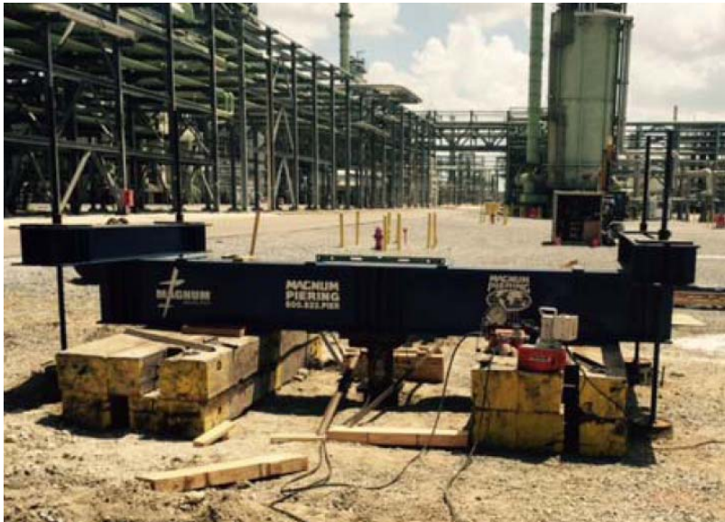
Figure 9- Compression Load Test (Courtesy of Magnum Piering, Inc.)
