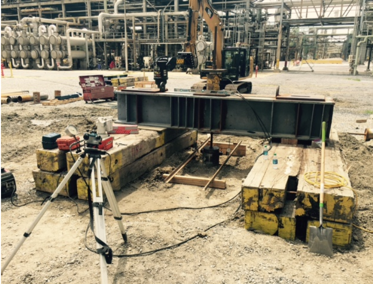
Figure 10- Tension Load Test (Courtesy of Magnum Piering, Inc.)
