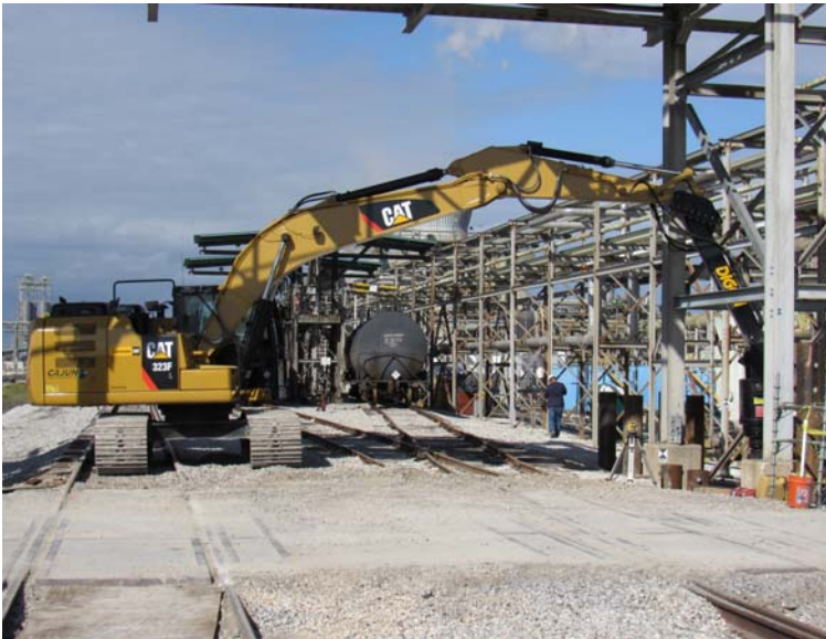
Figure 6- Limited Access Helical Pile Installation (Courtesy of Cajun Deep Foundations, LLC)
