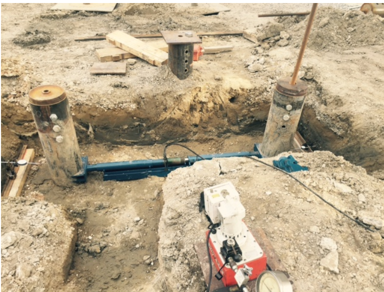
Figure 11- Lateral Load Test (Courtesy of Magnum Piering, Inc.)
