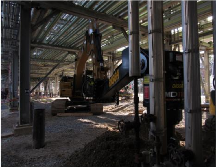
Figure 8- Confined Area Helical Pile Installation (Courtesy of Cajun Deep Foundations, LLC)
