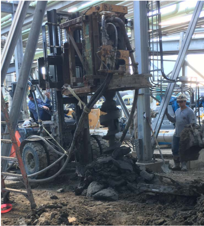
Figure 1- Low Overhead Auger Cast Pile Installation (Courtesy of ...)
